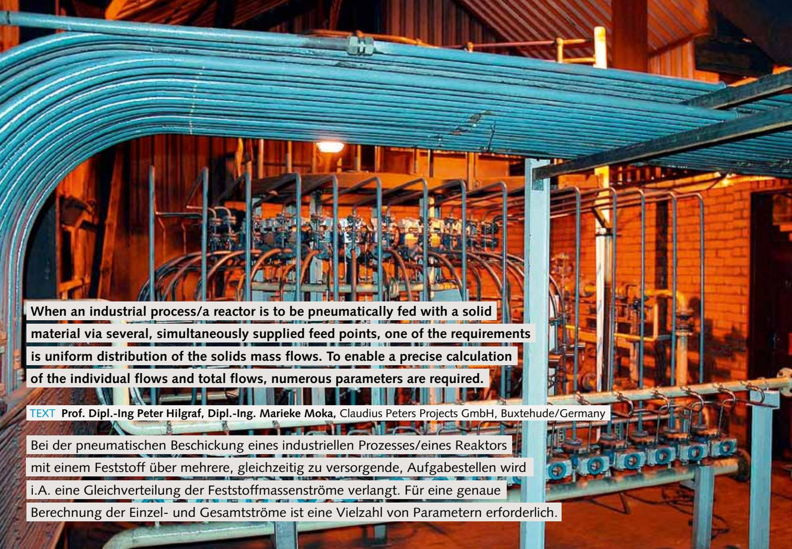
When an industrial process/a reactor is to be pneumatically fed with a solid material via several, simultaneously supplied feed points, one of the requirements is uniform distribution of the solids mass flows. To enable a precise calculation of the individual flows and total flows, numerous parameters are required.
