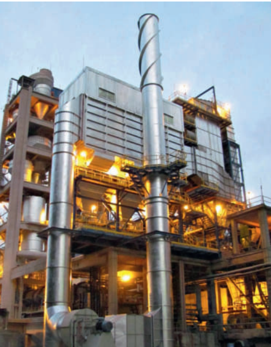
15 Clinker cooler bag filter
