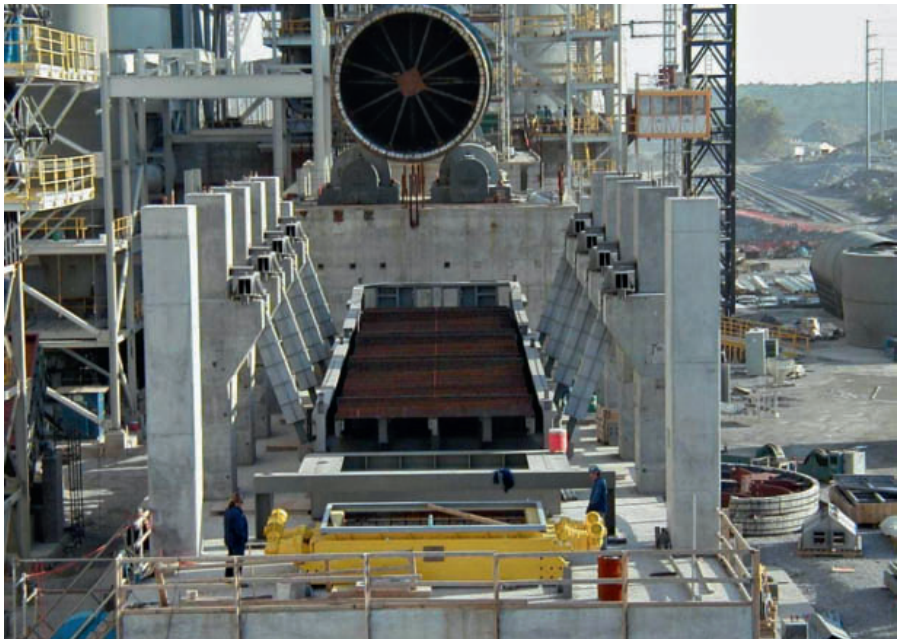
4 Erection of a Pendulum cooler
