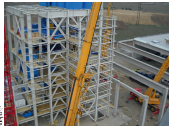
Building shell of the factory
