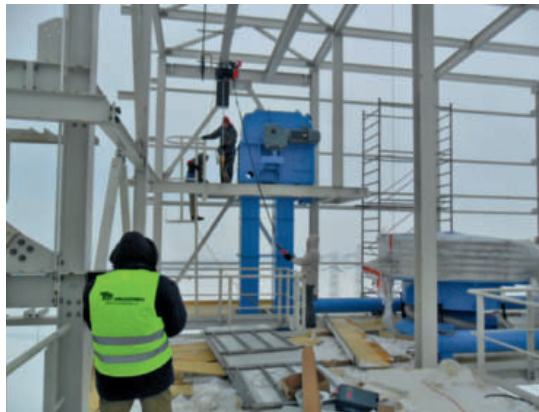
Installation of the plant components
