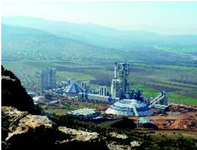
2 General plant view of KCS's Maras cement plant Ansicht des Zementwerks Maras von KCS
