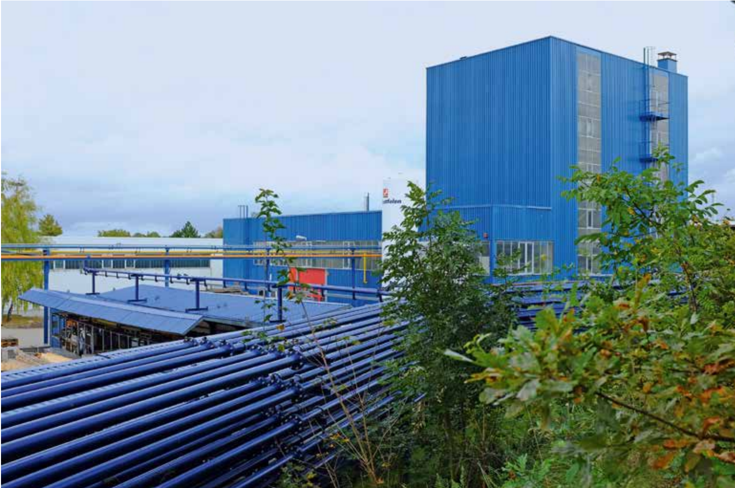
6 Modern test facility – 5 km long pneumatic conveying pipe
