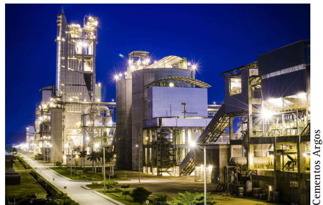
12 Cartagena cement plant in Colombia
