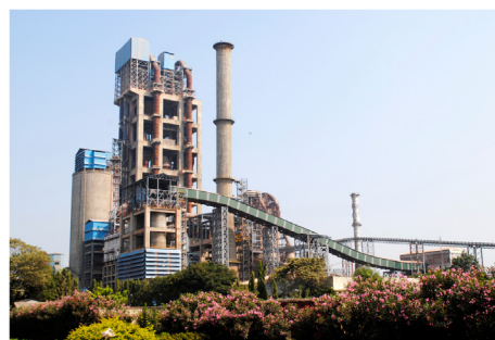
9 Manikgarh Cement Works
