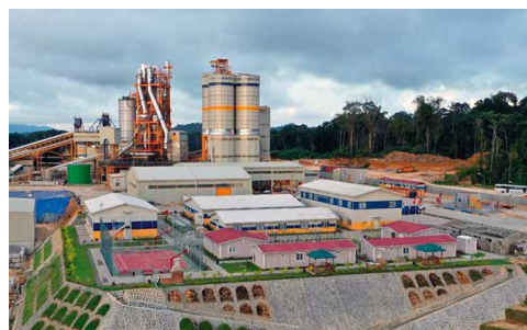
9 Kribi cement plant
