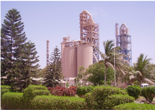
16 Hub cement plant
