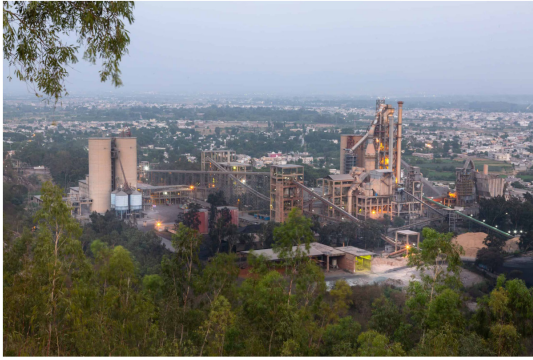
10 Wah cement plant
