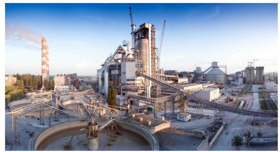
8 Karachi cement plant
