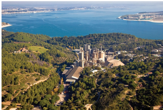
1 Photo: Integrated cement plant Outão in Portugal (Credit: Secil)
