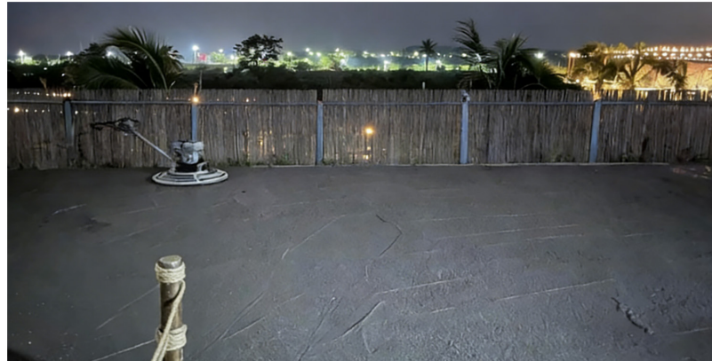
Figure 3 Nighttime placement and finishing operations of AAC under field conditions
