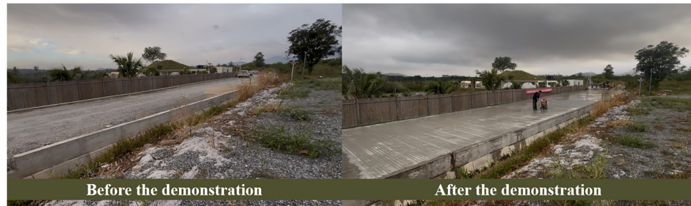
Figure 2 Field photograph of the completed pavement section at the demonstration site
