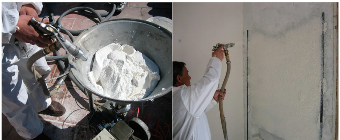
Figure 2 In situ application of the aerogel-based plaster [3]
