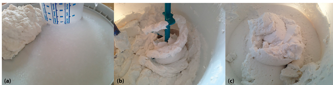
Figure 1 The direct mixing steps of aerogel with plaster: (a) original components; (b) mixing phase; (c) final composition of the plaster [3]
