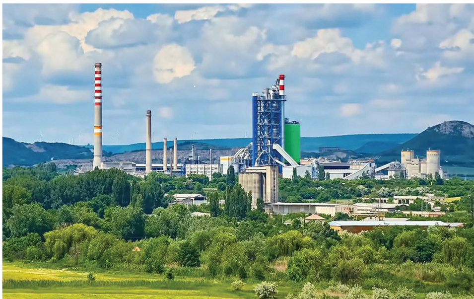
Figure 11 Devnya cement plant in Bulgaria (Heidelberg Materials)
