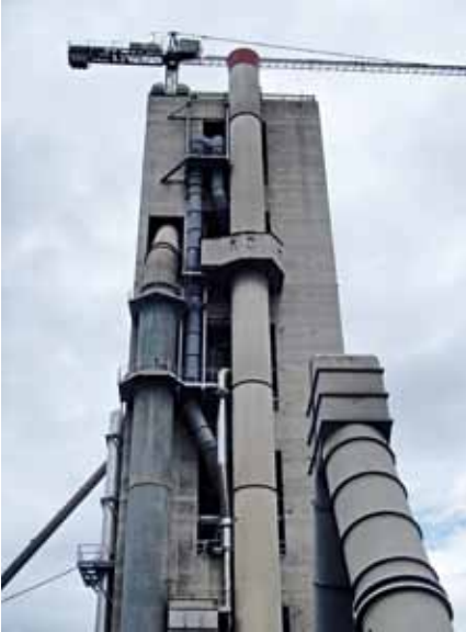
5 View of the second preheater line ductwork (between stack and downcomer duct)
