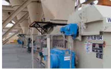
15 Weigh rail load cell mounted and Aumund weigh feeders at TXI Oro Grande
