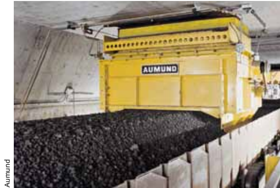
14 Clinker storage discharge
