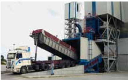
10 Samson material feeder – imported clinker intake
