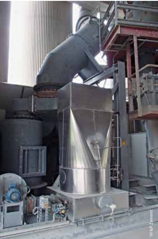
7 Partly visible cyclones for separation of the heated dust particles after the thermal treatment in the second preheater line
