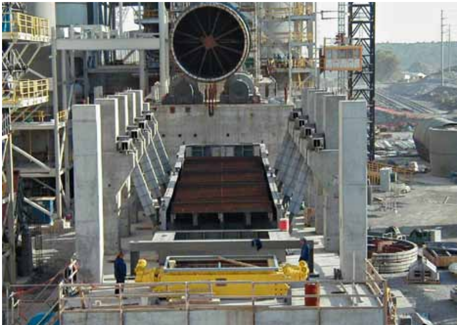
4 Erection of a Pendulum cooler
