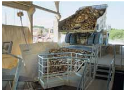
7 Off highway truck delivers mined minerals
