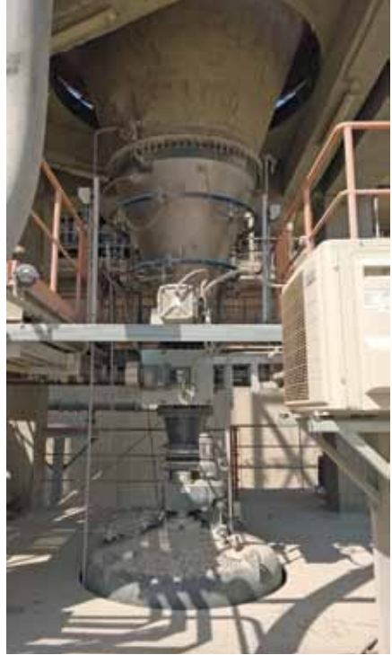
4 A closer look at the silo cone and pre-feeding devices
