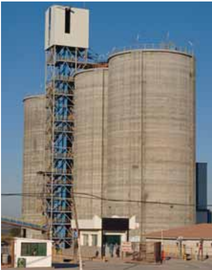
1 Aumund belt-bucket elevator type BWG
