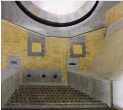
3 Static cooler grate
