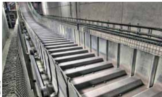
13 Clinker pan conveyor
