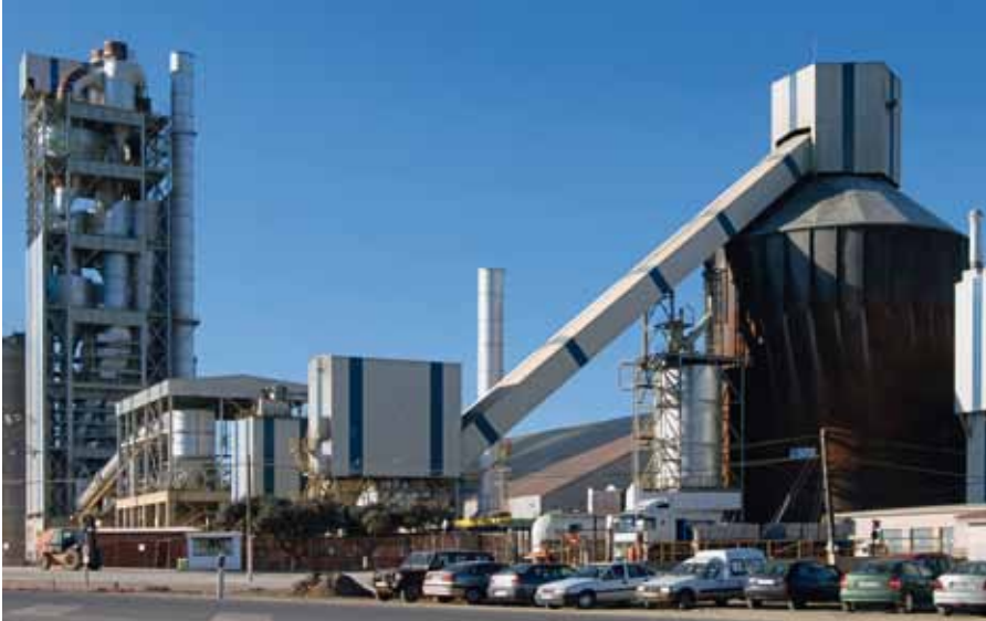
5 Upgrade to an Aumund BZB bucket conveyor
