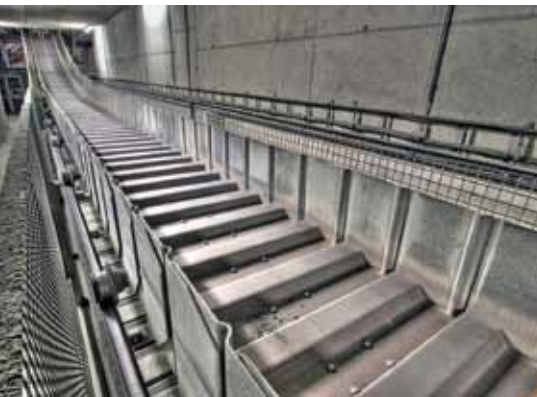
4 Clinker export – transport and silo and Aumund pan conveyor type KZB
