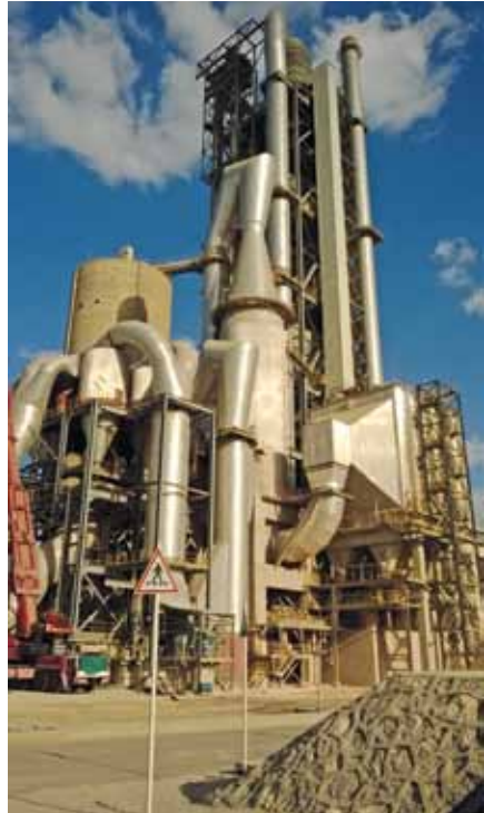
2 The calciner tower in Ain Sokhna
