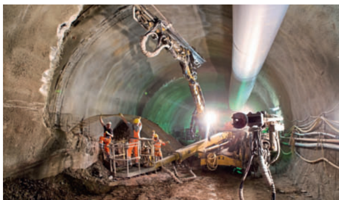
3 SikaRock is a hydraulically setting, purely mineral dry mortar. The SikaRock Anchor Mortar 1 variant in addition offers high protection against corrosion, while SikaRock Anchor Mortar HS is resistant to water containing sulphate
