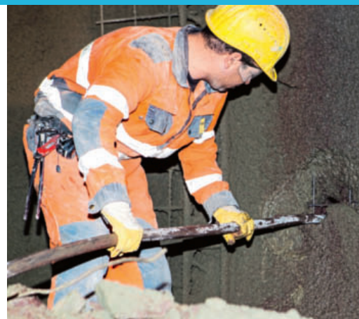
1 and 2 The two SikaRock Anchor Mortar 1 and SikaRock Anchor Mortar HS dry mortars are used for anchoring of rock nails and grouting/filling of rockbolt holes in mining and in tunnel engineering
