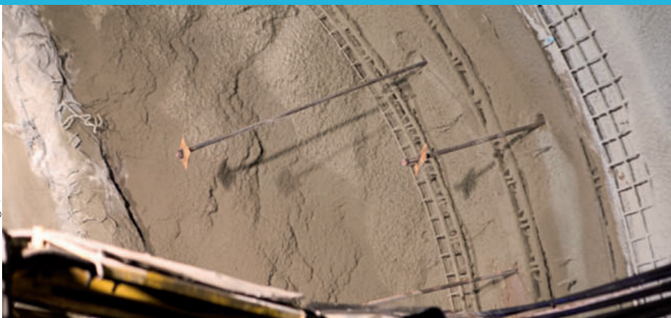
1 and 2 The two SikaRock Anchor Mortar 1 and SikaRock Anchor Mortar HS dry mortars are used for anchoring of rock nails and grouting/filling of rockbolt holes in mining and in tunnel engineering
